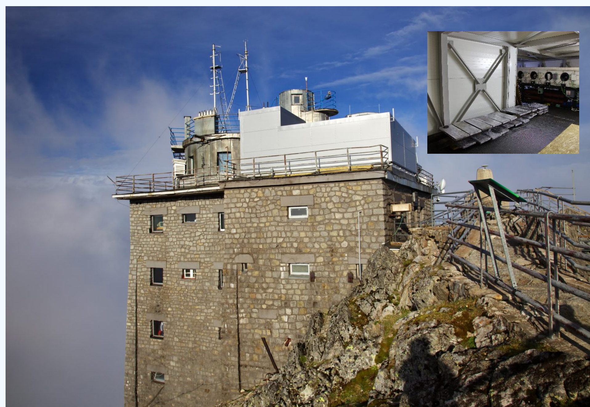
New container in order since June 30, 2012. SEVAN will be in the upper part on the left.
